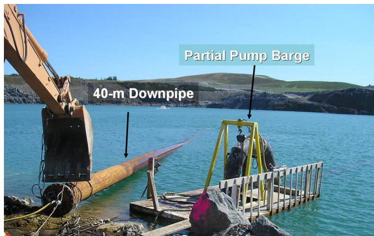
Figure 10: Deployment of Downpipe
